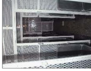
9-gauge expanded metal security walls and screening
