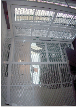
9-gauge expanded metal security walls and screening
