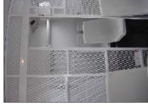
9-gauge expanded metal security walls and screening
